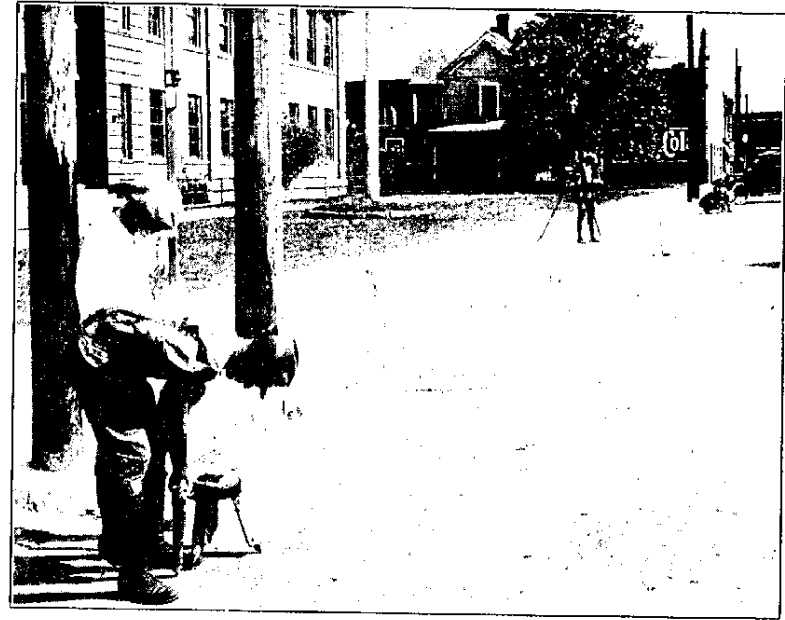
Fig. 7. Taping on Precise Traverse.
